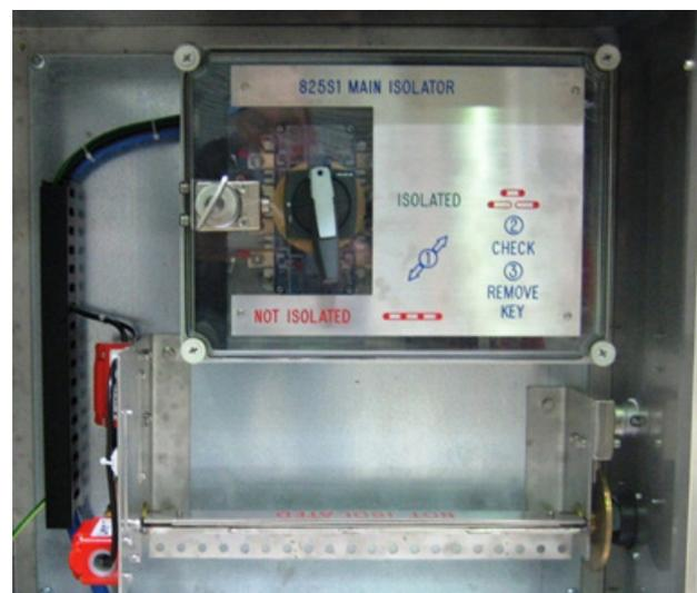
to ensure an effective isolation and incorporated Electrical, Electronic, Programmable Electronic (E/E/PE) components in its control system. With this being the case, the HIIS was designed, tested, installed and commissioned in accordance with the functional safety principles and lifecycle outlined in AS/NZS61508.
